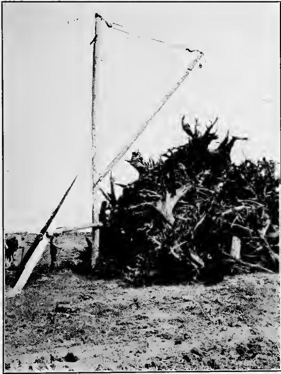
Fig. 62. Light Derrick Used on Tract 5
